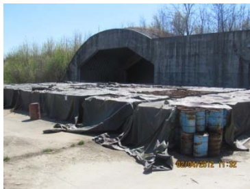
Stored at open space
